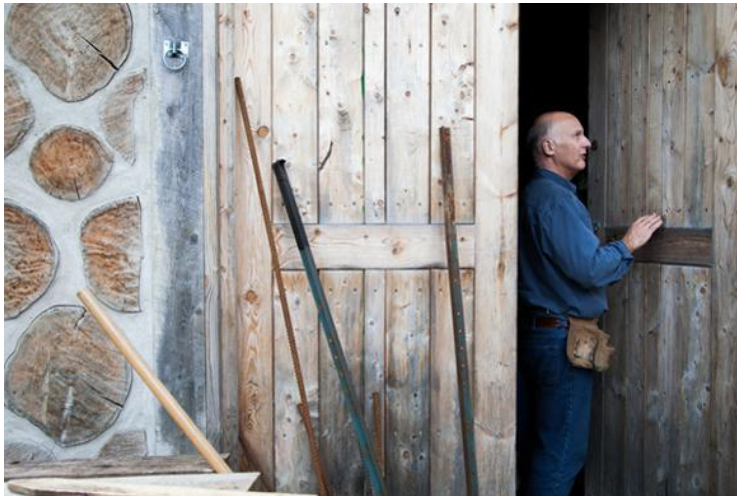
A builder works on an off-grid home in Quebec. Photo by Jonathan Taggart.
